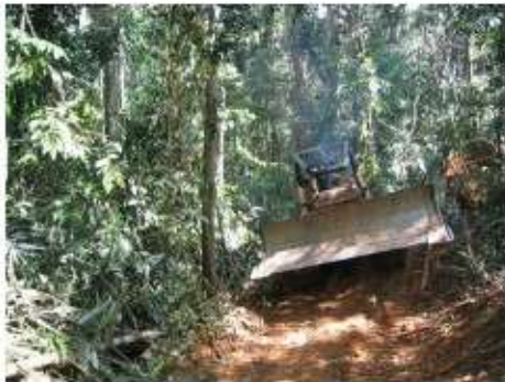
c. Opening of skid trail
