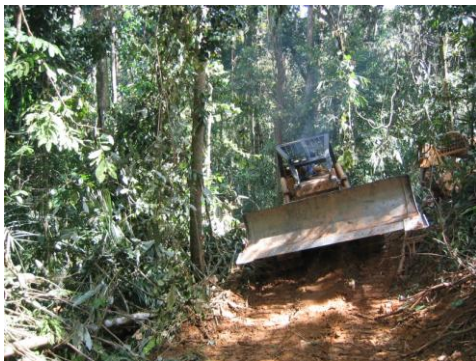
c. Opening of skid trail
